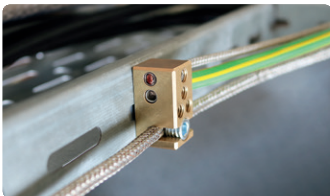
Fig. 13: Example for fastening of EMClots
