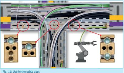
Due to the conductive structure of the terminal, metallic system components such as cable trays and pipelines are automatically integrated into the bonding system. Necessary wiring is reduced significantly.
